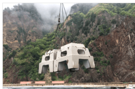
Installation of Triton artificial reefs
